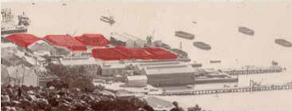
Figure 7: The Royal Navy's coaling station at Simon's Town, South Africa c.1900 – the huge piles of coal are highlighted in red.
