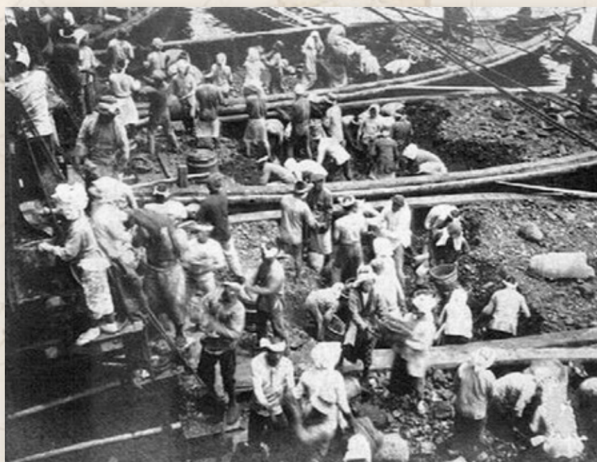
Figure 13: Three and a half coaling lighters, each carrying c.30 tons, can be seen with c.69 labourers shifting coal, so an average crew-per-lighter of 20 c.1900.
